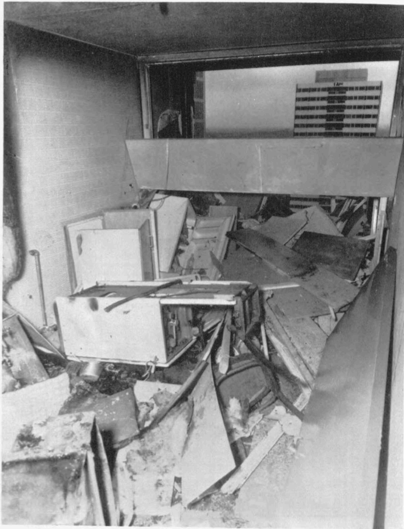
Plate No 7 Miss Hodge's gas cooker showing the flexible hose
